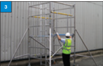
3. Fit the BoSS Cam-Lock Advance Guardrails.
