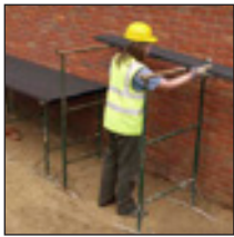
Steel Trestles & Scaffold Boards
