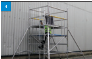
4. Fit the decks. To build higher - simply repeat steps 2, 3 and 4.
